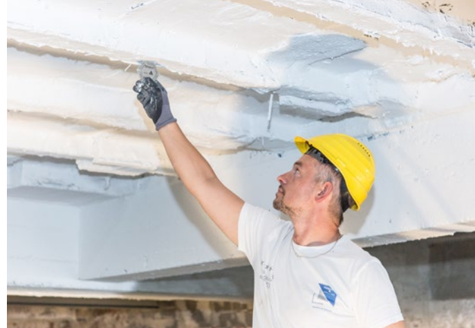
Measurement of the wet film layer thickness directly after the application.
