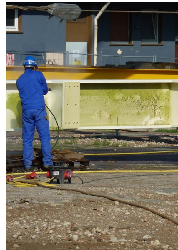
High-pressure cleaning of the steel beams
