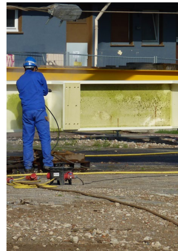
High-pressure cleaning of the steel beams
