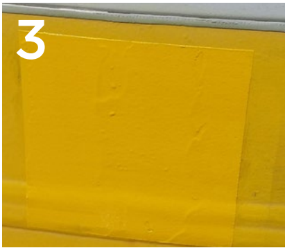
Repaired, reconditioned surface is cured after just a few hours
