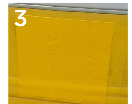
Repaired, reconditioned surface is cured after just a few hours
