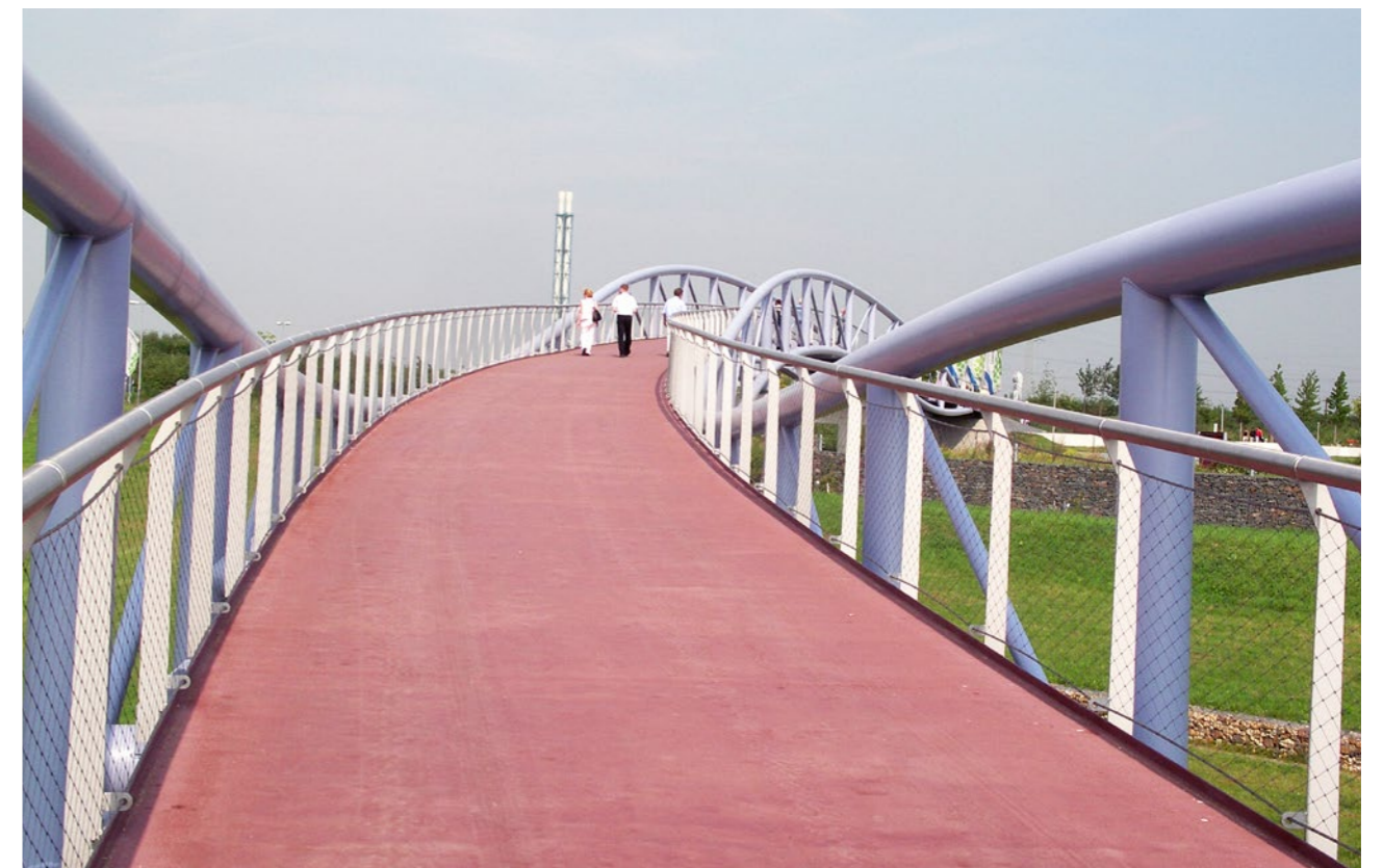
Pedestrian and cycle path bridge Leverkusen, Germany, 2005
