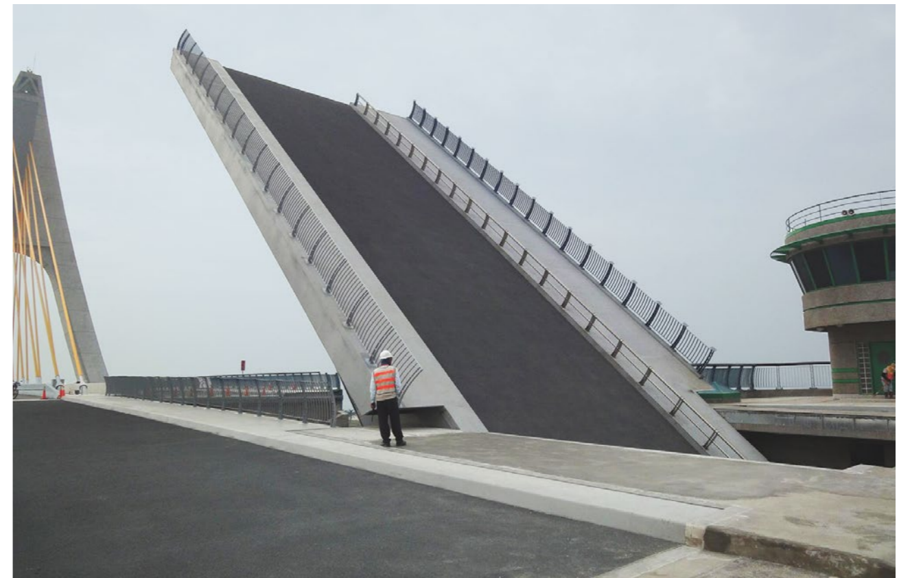
Steel bascule bridge Donggang, Taiwan, 2011
